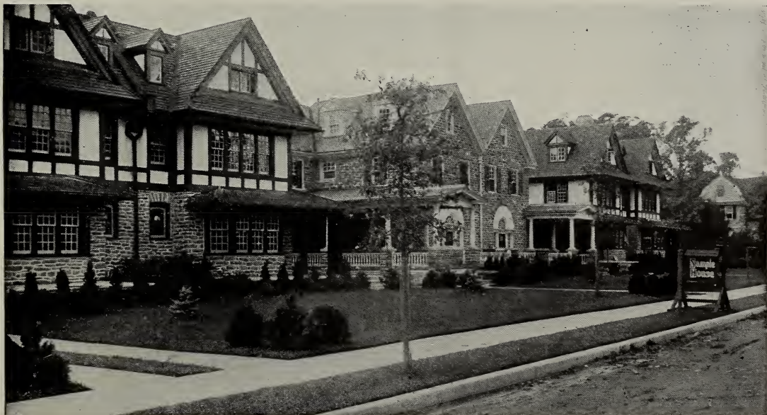
Here is an illustration where a very clever building operator clothed his proposition in a good suit, —or shall we say, “framed his picture.”
